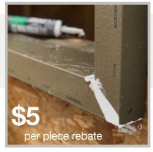
ThermalBuck solves the challenge of installing windows with exterior insulation. Choose from 7 different depths from 1" - 4", priced per 8' length. Works with all types of exterior insulation. Backed by a 15 year warranty.
