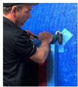
Wrap the face flap of tape along the side of the ThermalBuck at jambs and on to the sheathing. Bring the second flap down along the side of the jamb, for a shingle effect.
