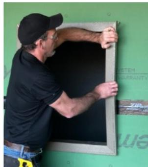
Repeat for each jamb and head piece, considering which one will be easiest to flex into place last. Ensure all corners align before nailing tongue, and adjust as needed.
