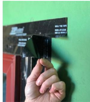
Wrap the face flap of tape along the side of the ThermalBuck at jambs and on to the sheathing.
