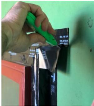
Make two horizontal cuts in the tape, following the lines of the ThermalBuck.
