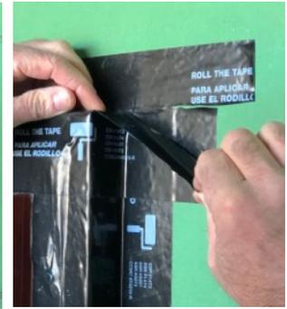
Bring the second flap down along the side of the jamb, for a shingle effect.
