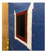
Release head flap over head flashing tape.
