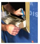
Cut jambs and sill flush with outside edge of ThermalBuck.
