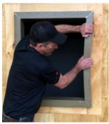
Repeat for each jamb and head piece, considering which one will be easiest to flex into place last. Ensure all corners align before nailing tongue, and adjust as needed.
