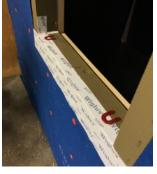
Cut tape at face of jamb legs, and fold up past interior corner and across outside face of jamb and WRB.
