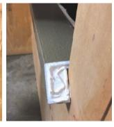
SEAL ENDS Add sealant to mitered ends.
