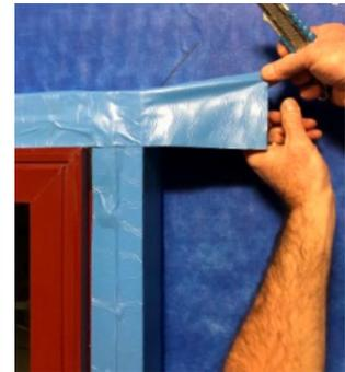
Make two horizontal cuts in the flashing tape, following the lines of the ThermalBuck.
