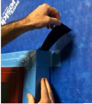
Wrap the face flap of tape along the side of the ThermalBuck at jambs and on to the WRB.
