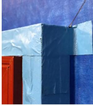
Bring the second flap down along the side of the jamb, for a shingle effect.
