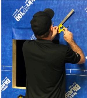
Angle cut head corners 6", and sill corners 4" away from RO.
