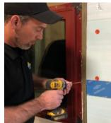
Adhere the tape from sill down and over the ThermalBuck and onto the insulation.
