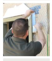
Flash entire length of each jamb, extending 2" past ThermalBuck on top, and 4" on bottom. Flashing should cover both ThermalBuck and WRB.
