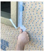
Cut end of flashing in half lengthwise to continue 90° angle. Press the outer half against the structure. Press the inner half against ThermalBuck, wrapping around the corner.
